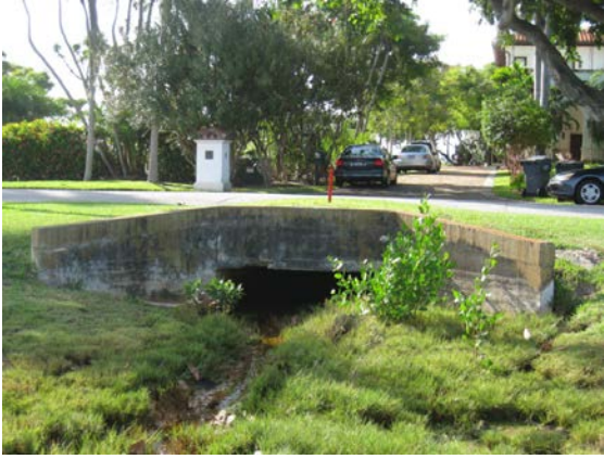
Photo 5: Channel Inlet 1 with Headwall
