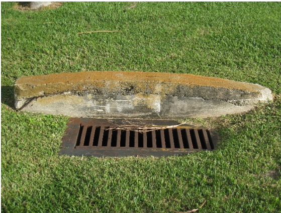
Photo 7: Grated Inlet 5A with Headwall
