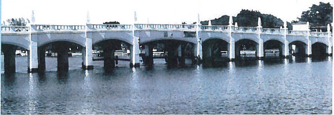
The Indian Creek Bridge provides access to the island community of Indian Creek in Miami-Dade County.
