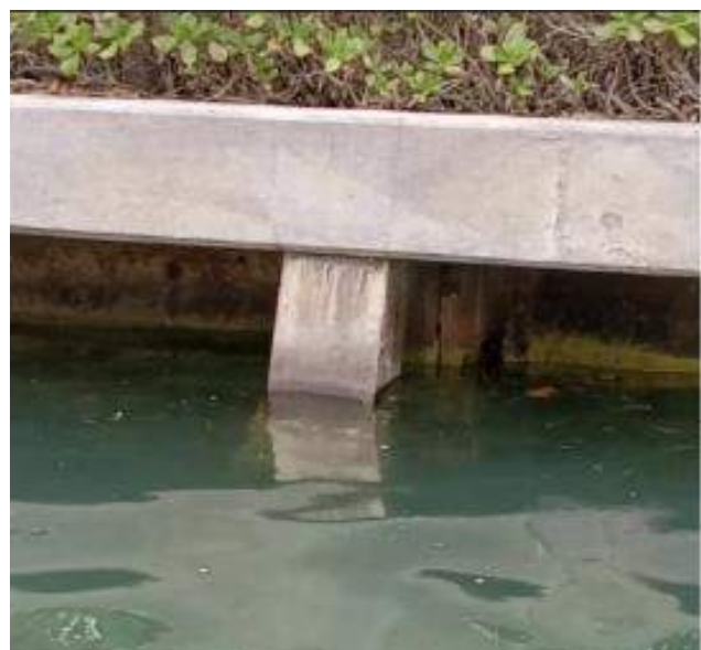
Figure 14: Vert. Encasement Spall @ Several Locations
