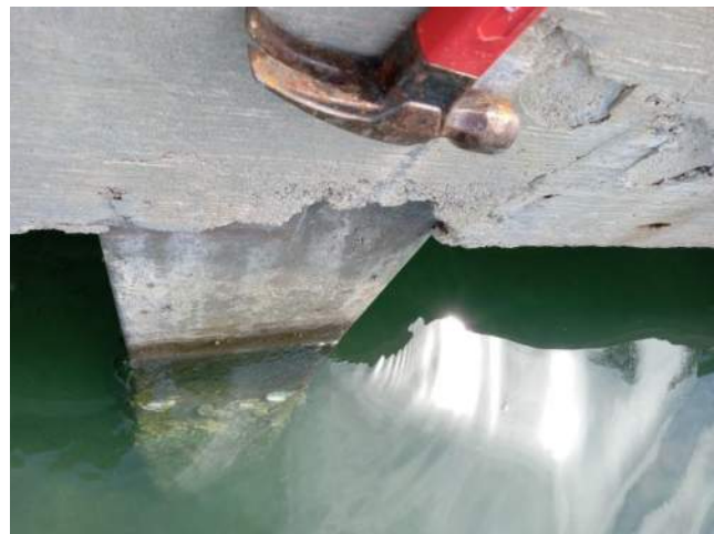
Figure 10: Delamination @ 90' from N. End
