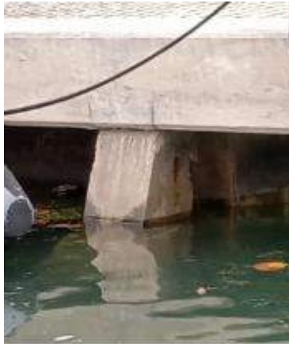
Figure 15: Prestressed Battered Pile Spall on Inner Side
