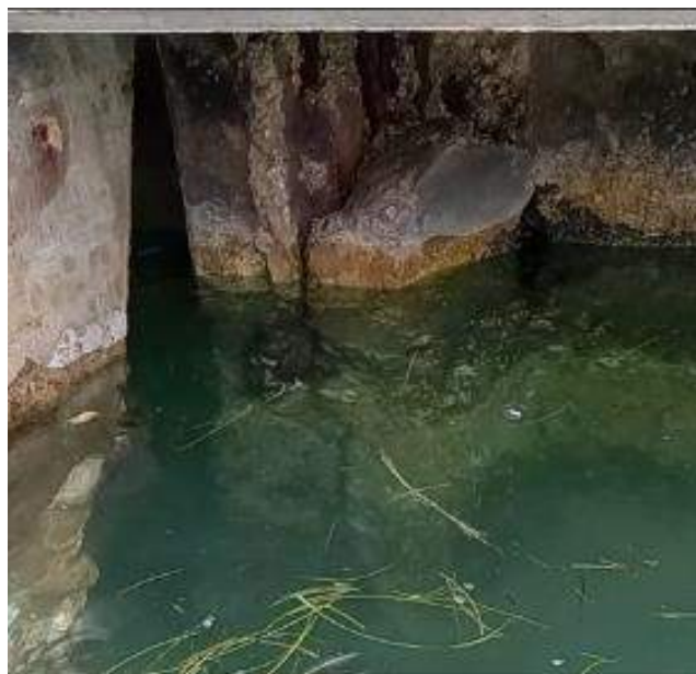
Figure 12: Vert. Encasement Spall @ 45' from S. End
