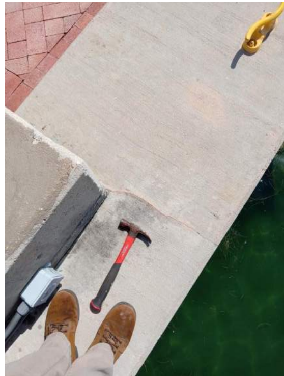
Figure 8: Delamination @ 50' from N. End
