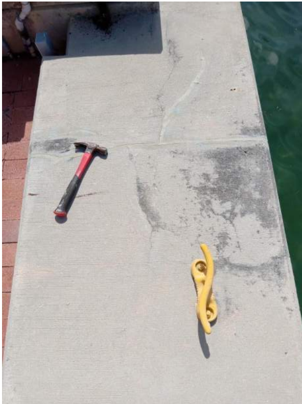
Figure 9: Delamination @ 70' from N. End
