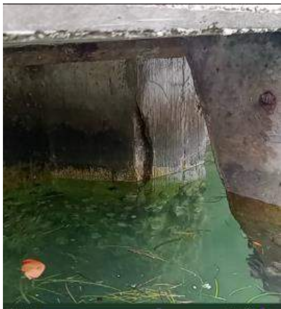
Figure 13: Vert. Encasement Spall @ Several Locations
