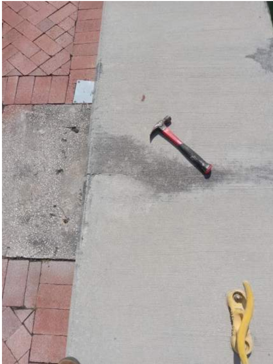
Figure 7: Delamination @ 30' from N. End
