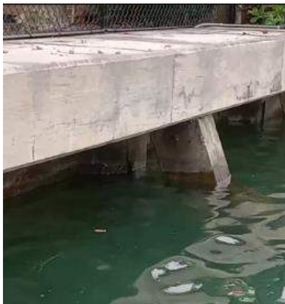
Figure 11: Vert. Encasement Spall @ 15' from S. End
