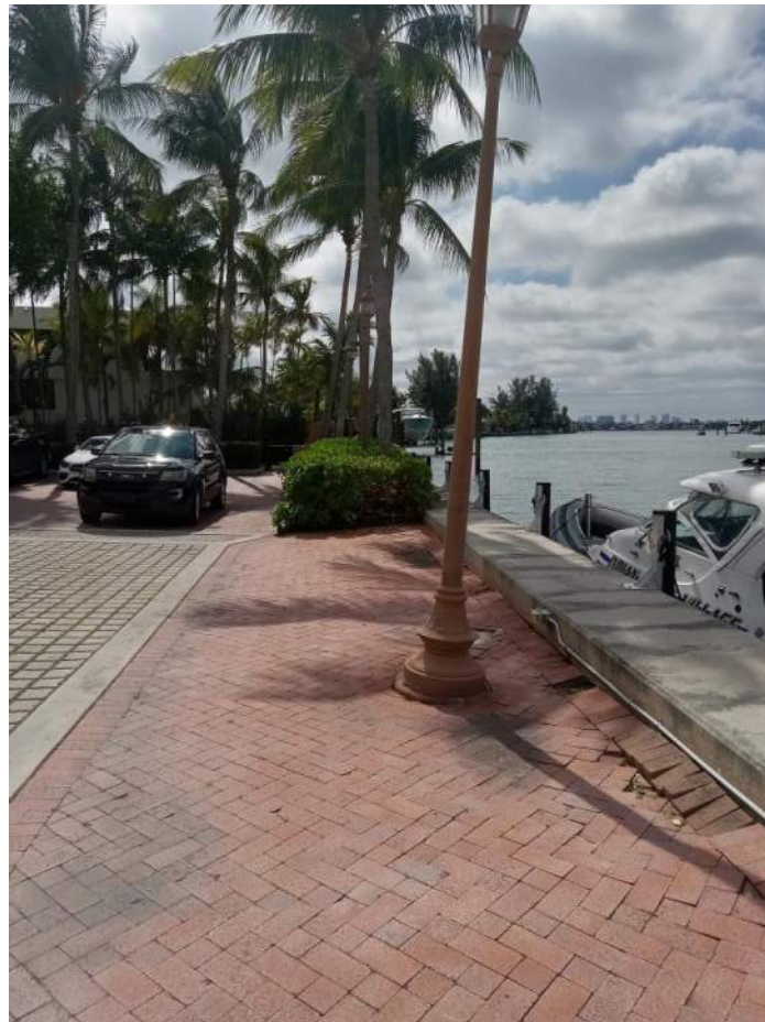
Figure 1: Ground Subsidence
