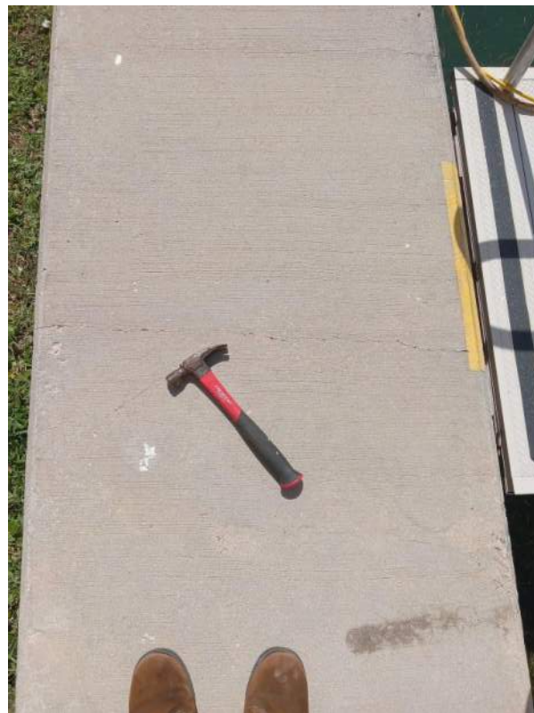
Figure 6: Typical Cap Shrinkage Crack @ 4' C.C.
