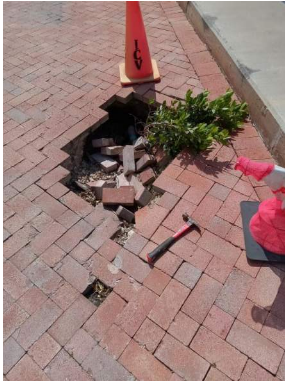
Figure 4: Paver Caving
