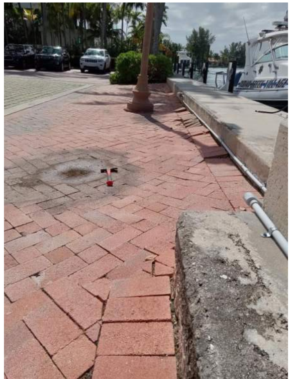
Figure 5: Ground Subsidence
